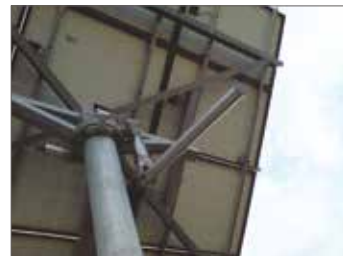
Inspection from the back shows no hot spots, the hot spots in the previous thermal image taken from the front were caused by cloud reflection.
