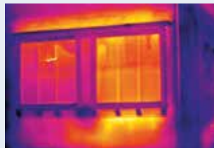
What a thermal imaging camera sees.
