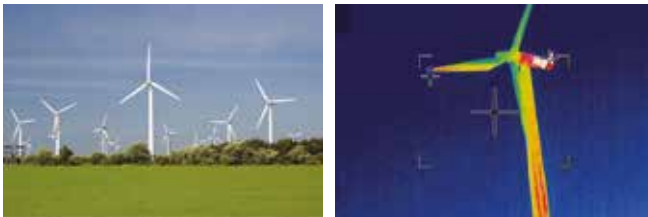
A thermal image of a wind turbine taken from ground level
